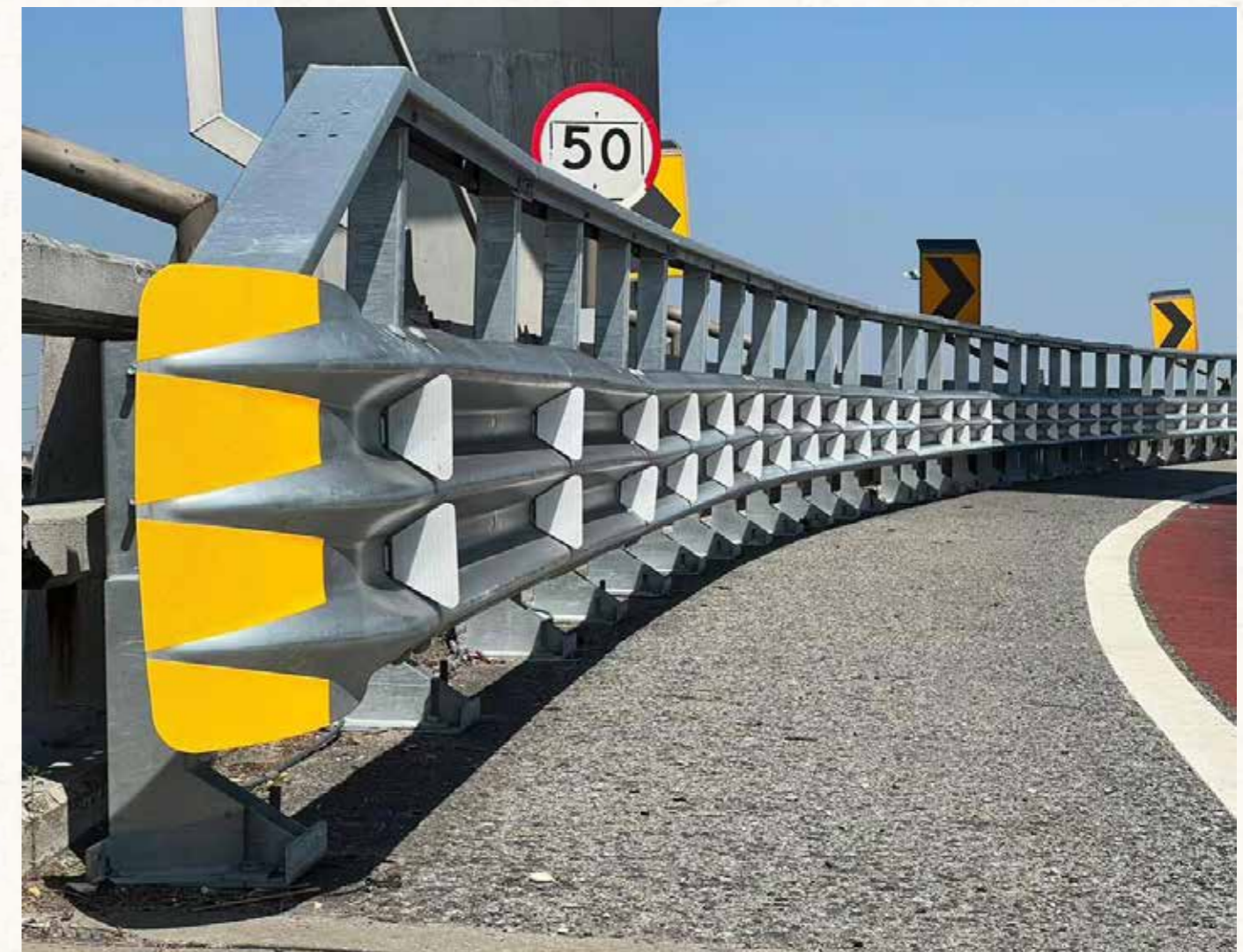
Safety barriers and guardrail
